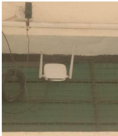
Department of Chemistry Wifi F23F-MTC, Dnyaneshwargar, Maharashtra 414605, India Lat: 19.4335281 / Long: 75.022998 Friday 16 February 2024 10:49:34
